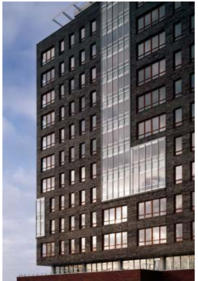
▲ Enschede, Twentec project
